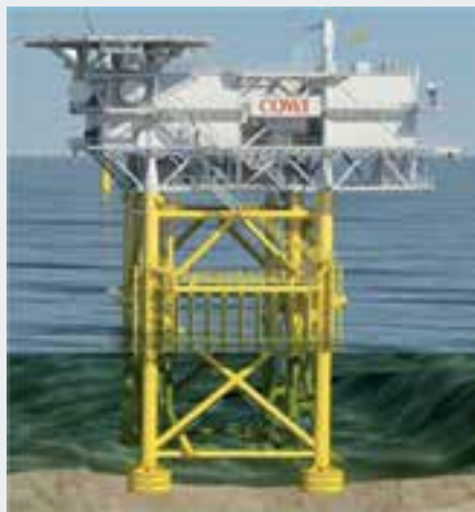
FIGURE 15-6 OFFSHORE SUB STATION FOR A EUROPEAN OFFSHORE WINDFARM
